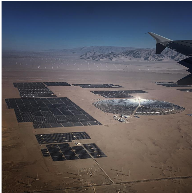
50MW Concentrated Solar Power Plant in Golmud, Qinghai Province
